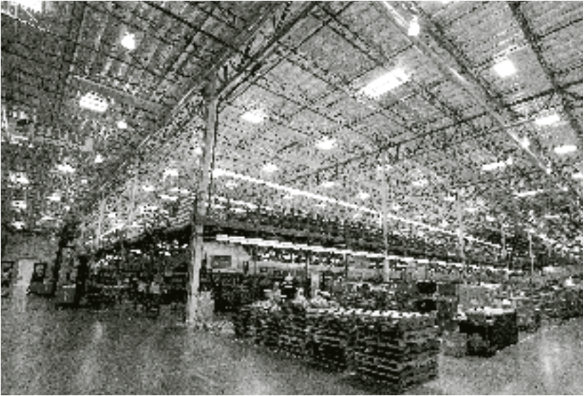
Skylights that track the sun and translucent roof-mounted smoke vents provide natural light, which reduces energy use and increases worker productivity. PHOTO: TIM DAVIS
