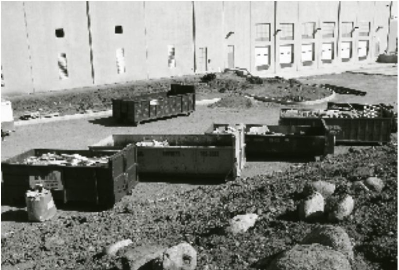
Construction waste – including metal, concrete, cardboard and wood – was separated for recycling. PHOTO: JANE DAY
