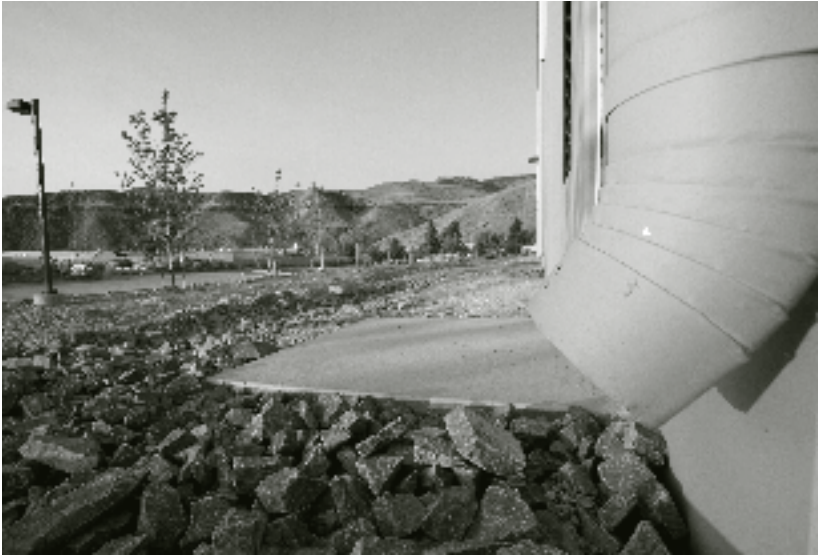
Rain and snow that falls on the roof, parking lot and walkways is directed to permeable surfaces and into the soil, which filters out contaminants. PHOTO: TIM DAVIS
